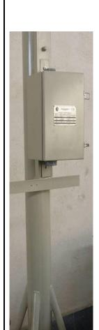
Permanent Test Stations are provided at selected locations along the protected structure to check, monitor and control the performance of cathodic protections.
