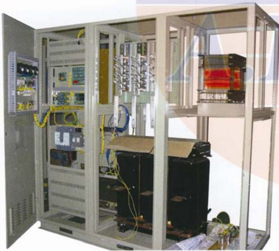
View of Rectifier Assembling Works
