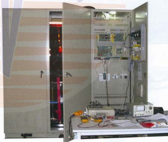
View of Rectifier Testing
