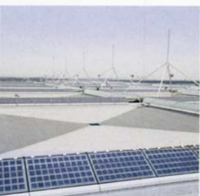
10 Aviation directional lighting
